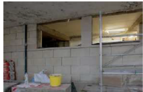
General View: front elevation.
