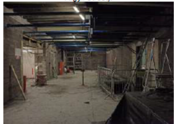
General View: Club / Venue (looking West).
