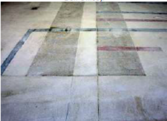
General View: Main Entrance terrazzo flooring exposed.
