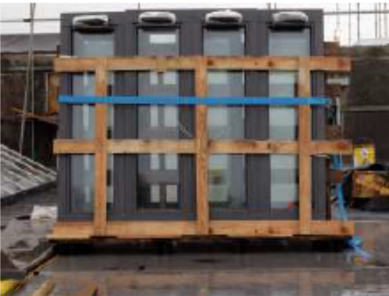
Auditorium Roof Light: patent glazing.
