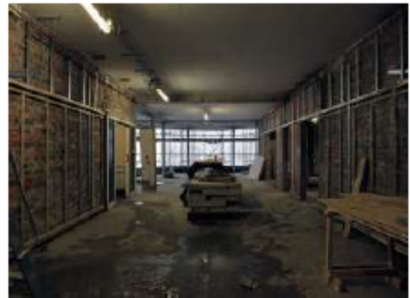
General View: new Café/Kitchen area.
