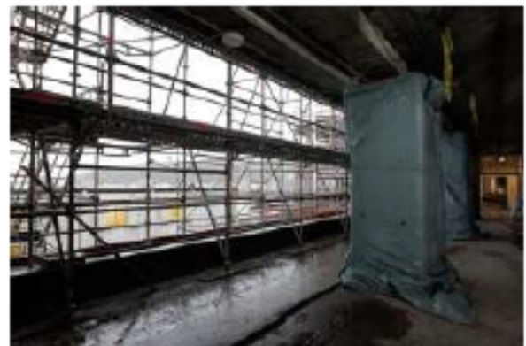
General View: Auditorium East wing.
