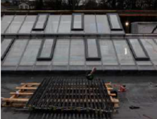
Looking West: new patent glazing to Auditorium roof light.
