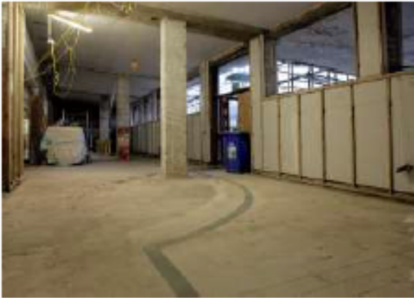
General View: New Exhibition area front wall.
