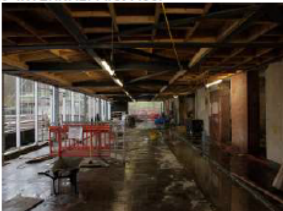
New Offices: General view A (looking West).
