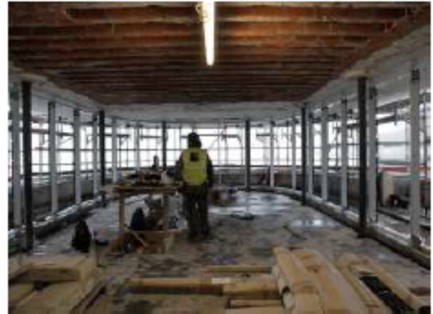
New Exhibition/Function Space: Looking East (towards Argyll St.)
