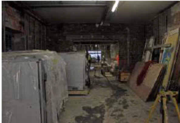
General View: reverse view looking out of Café towards main Staircase.
