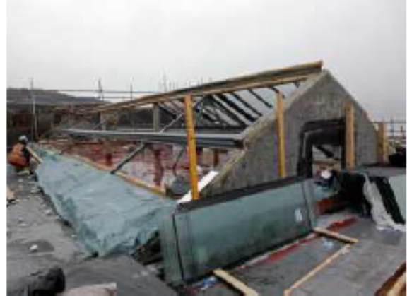
Looking (facing Mackinlay St): new steelwork to the roof light (NB: temporary waterproof protection partially removed).
